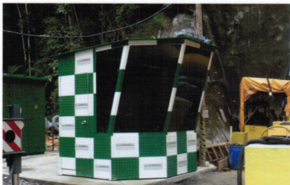
Roller System Control Cabin
