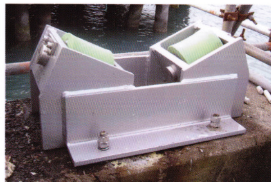
View of roller applied to pier
